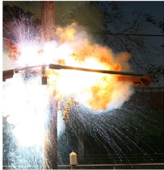
Fig. 1. A staged arc flash test.
