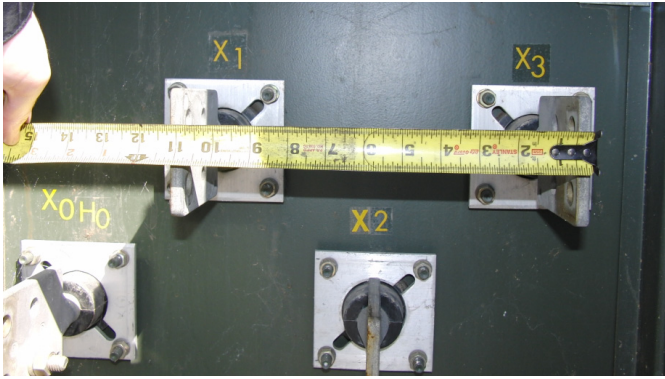
Fig. 10. 480-V padmounted transformer secondary terminals
