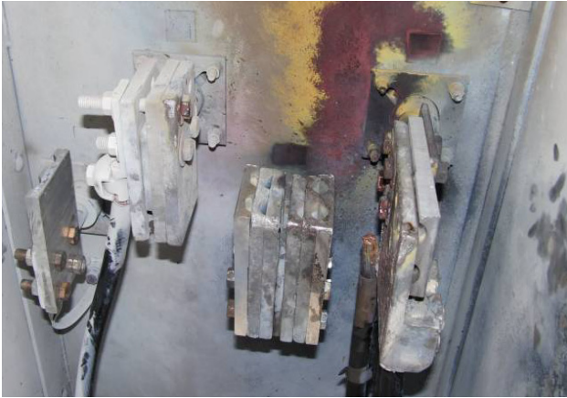
Fig. 16. Event 317: two-inch gap between phases
