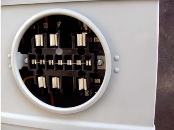
Fig. 9. Shorting wire in the meter base
