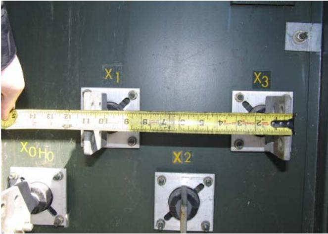
Fig. 13. 480-V padmounted transformer secondary terminals
