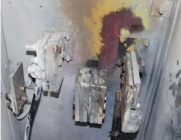
Fig. 20. Event 317: two-inch gap between phases
