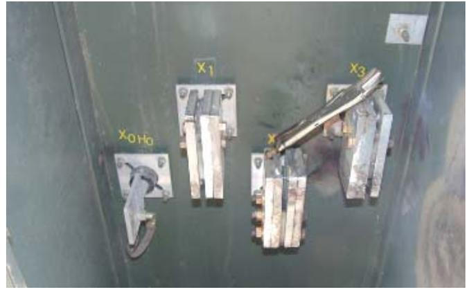
Fig. 14. Vice grip initiated test setup
