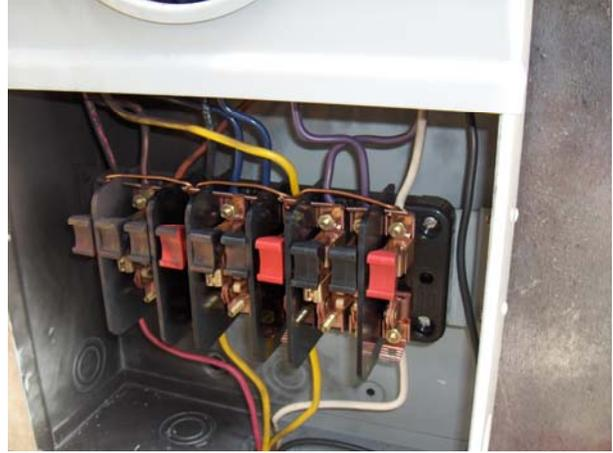
Fig. 10. Shorting wires in the switch block
